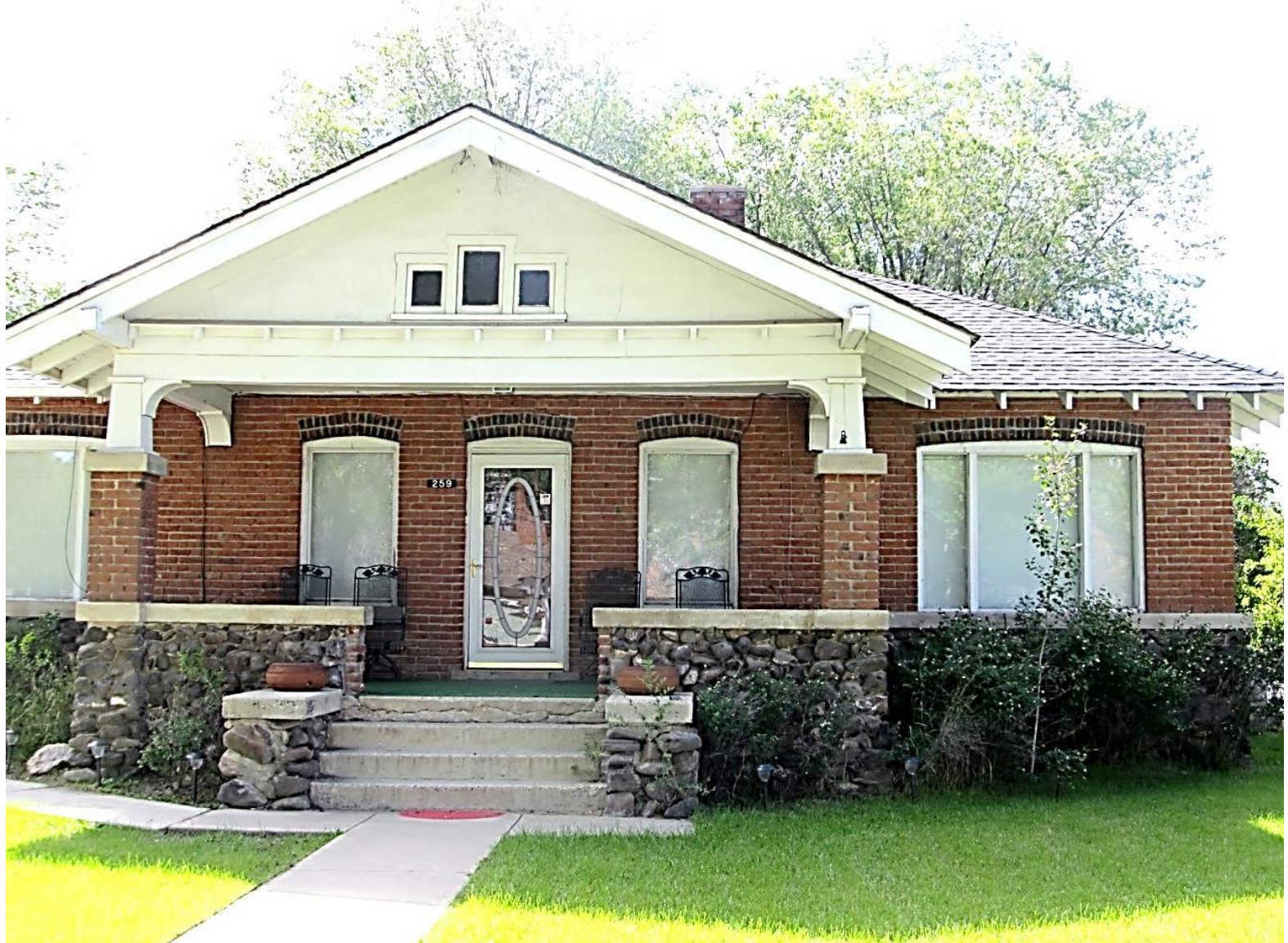
Brick Home built in 1918 by Dewey and Pauline Clark 259 North Main Craftsman Bungalow Style Note the exposed rafters and rock porch
