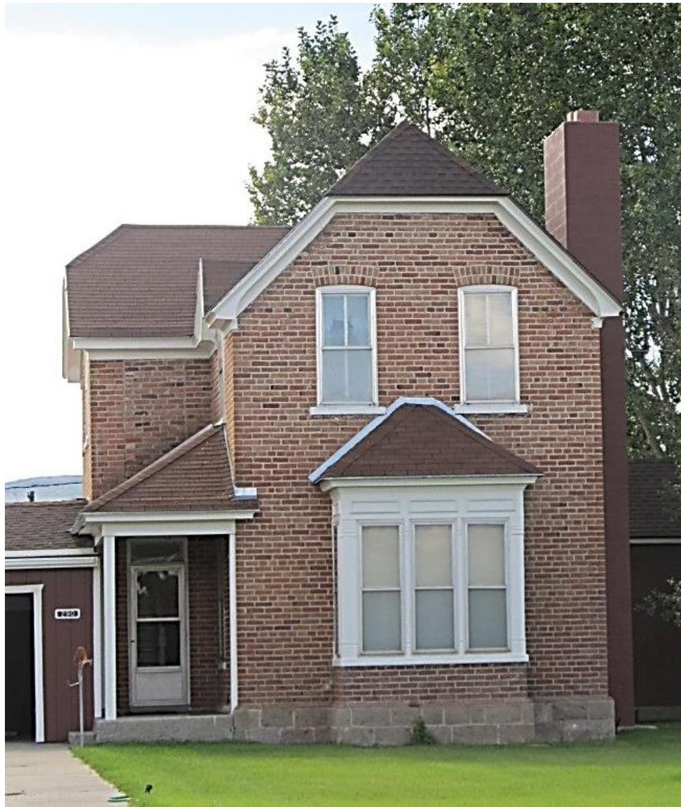
Brick home built in 1900 by George and Sarah Dodds 290 South 100 East Victorian Eclectic Style, Crosswing plan Note the bay window and varied colors of brick
