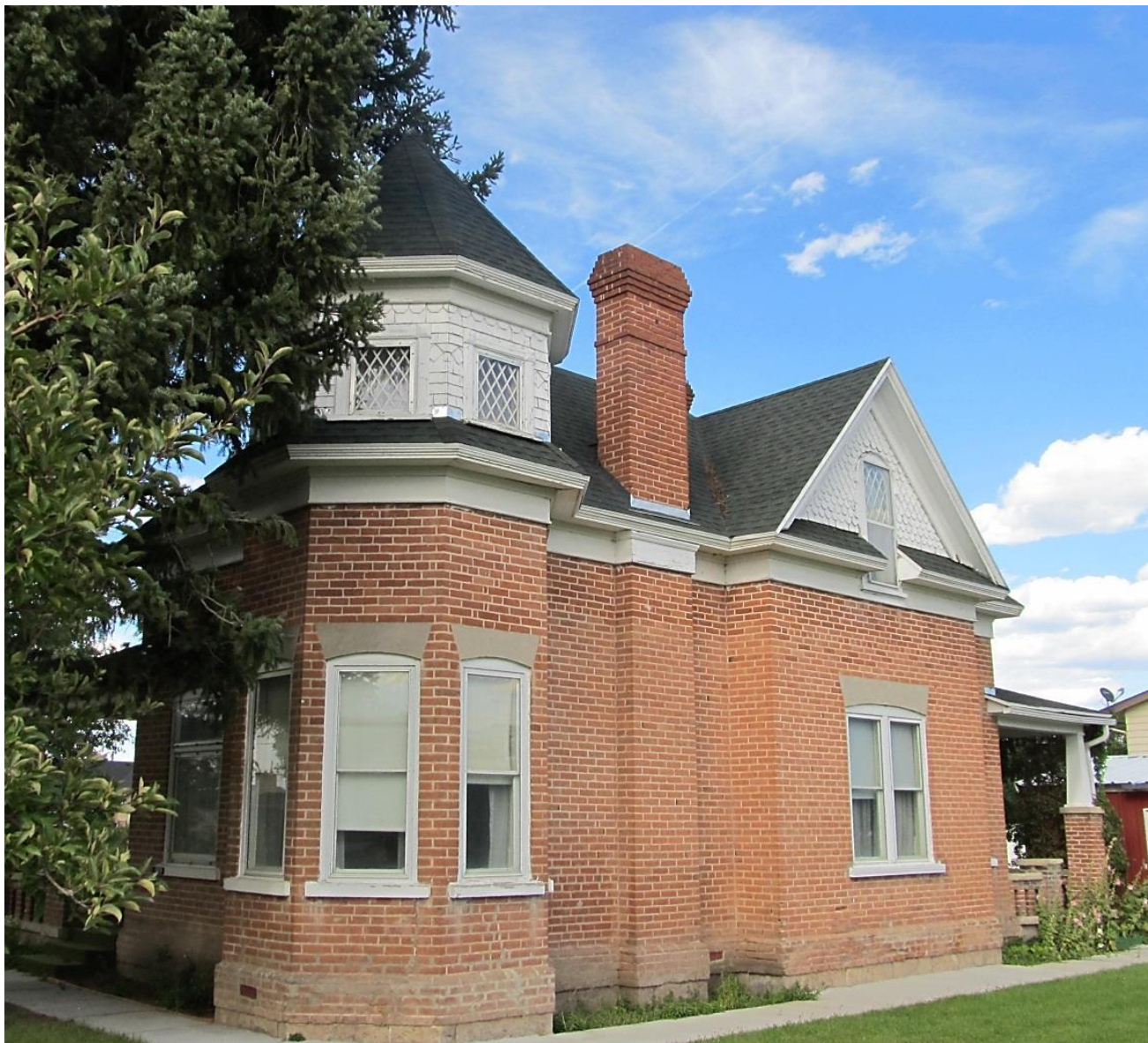
Brick home built in 1905 by Joseph and Margaret Heywood 182 South 200 East Queen Anne Style Note the shingles on tower and gables
