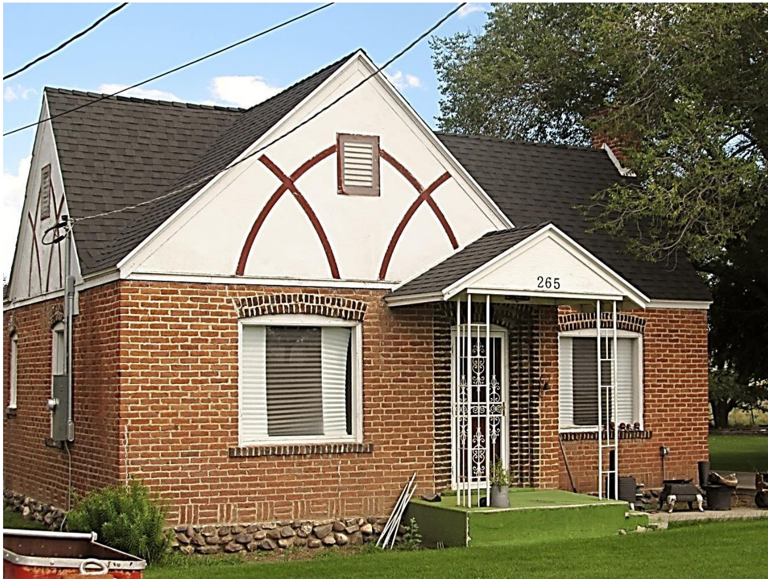
Brick Home built in 1936 by Alfred and Clea Cherrington 265 South Main Bungalow Style Note timber design and clinker brick window detail
